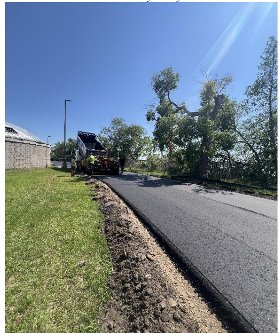
Figure 8: Friday, August 15 th , freshly paved asphalt on south access road.
