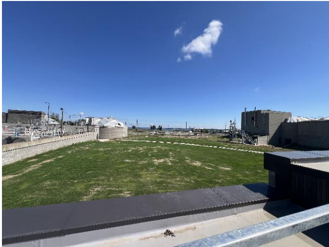
Figure 9: Thursday, August 28 th , roof view of newly seeded area growing.
