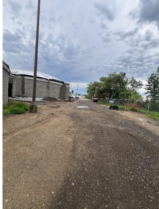
Figure 2: Friday, August 8 th , exterior view in front of new secondary clarifier.
