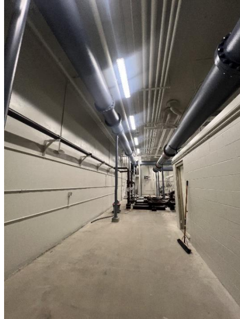
Figure 14: Thursday, July 24 th new paint inside new secondary gallery.
