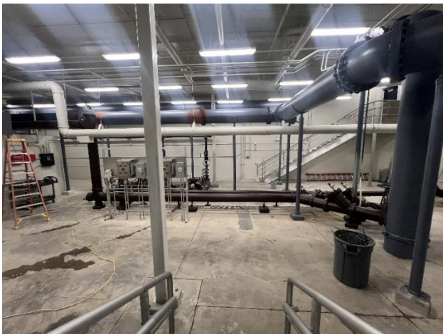
Figure 15: Thursday, July 24 th cleaned up site of new secondary gallery.
