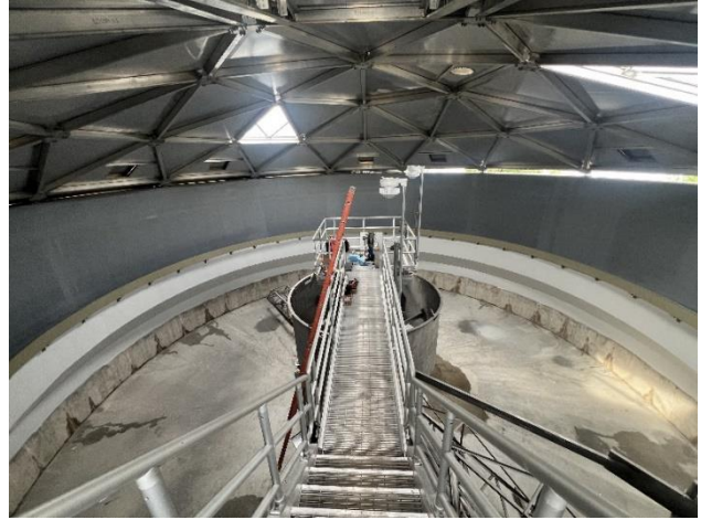
Figure 6: Thursday, July 10 th view inside new secondary clarifier.
