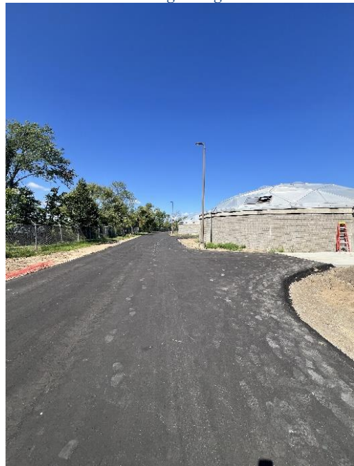
Figure 12: Thursday, August 28 th , view of south access road.
