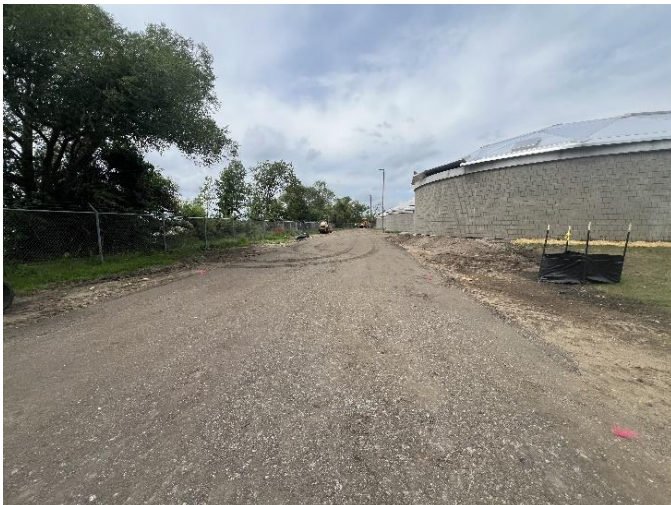
Figure 7: Thursday, August 14 th , freshly proof rolled south entrance road.
