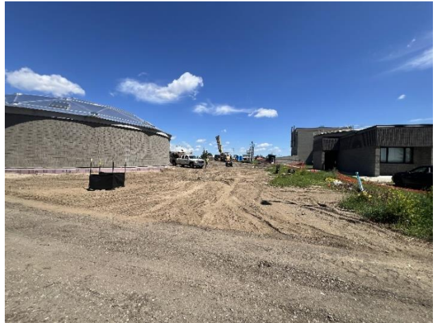
Figure 2: Tuesday, July 1 st exterior view in front of new secondary clarifier.
