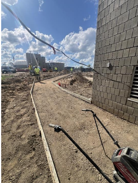
Figure 9: Thursday, July 17 th formed up sidewalks before pour.
