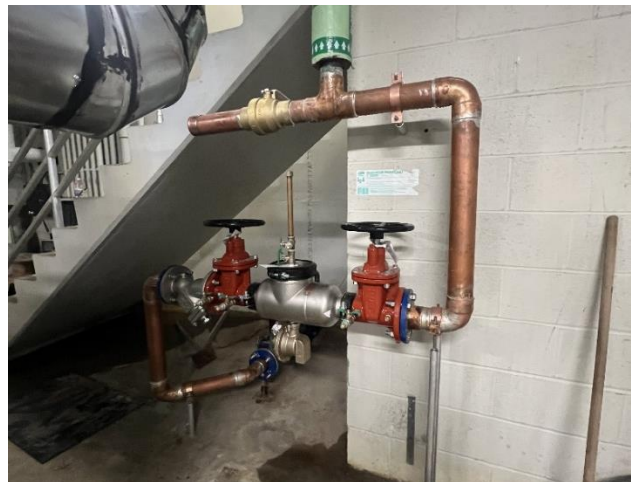
Figure 16: Thursday, July 24 th new RPZ in existing secondary gallery.
