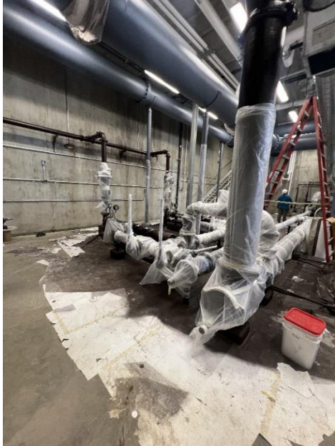
Figure 5: Tuesday, July 8 th interior of new secondary gallery, process pipes coated.
