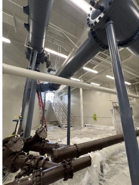
Figure 10: Thursday, July 17 th fresh paint inside new secondary gallery.
