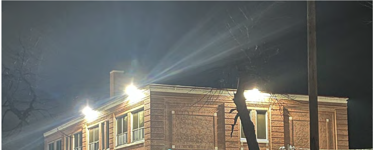
Exterior lighting violations, February 4, 2026.
